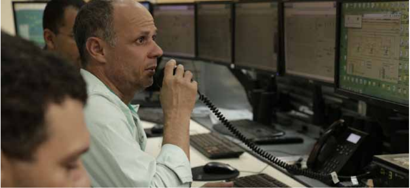
Geraldo Farias Distributed control system operator Drying
