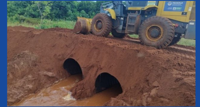
Donation of HDPE pipes for maintenance of a bridge providing access to rural residents, in partnership with the Municipality of Inocência.
